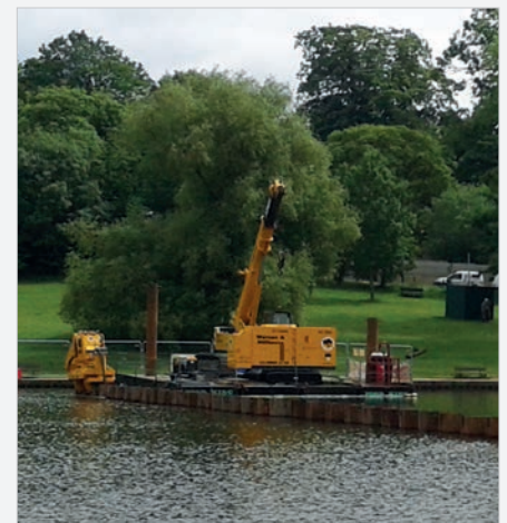
Work over water
