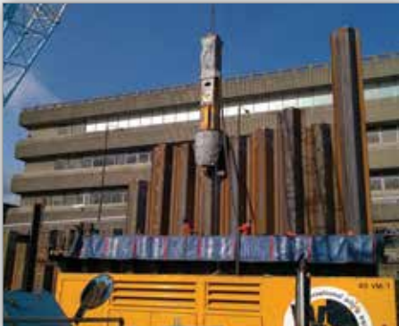
BSP CX85 hammer, fitted with acoustic shrouding, installing sheet piles
