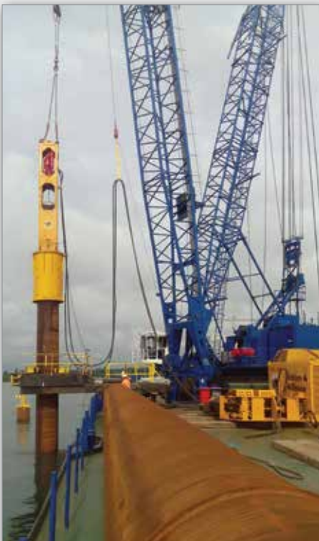
BSP CG300 driving tubular piles
