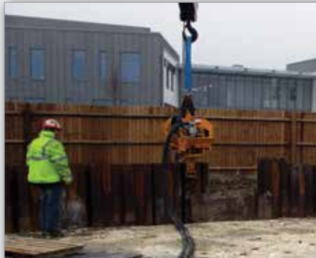
Crane suspended OMS OVR S-50 extracting sheet piles
