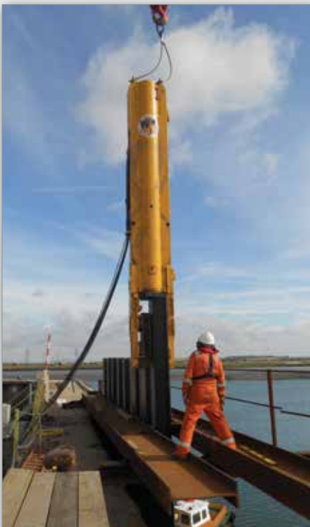
BSP SL30da installing sheet piles
