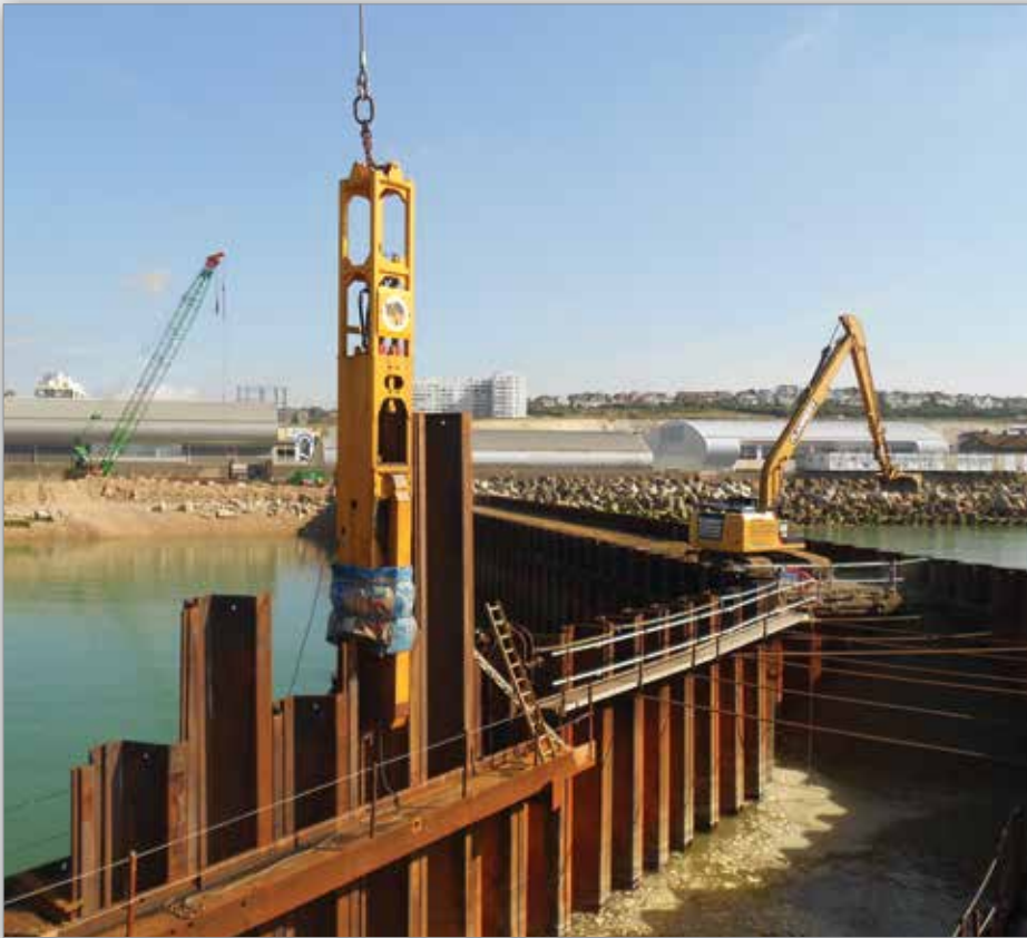
The newly introduced BSP CX579 installing sheet piles to create a cofferdam
