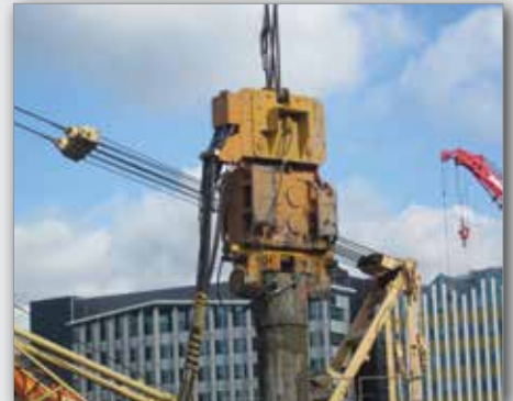
PVE 2319VM, fitted with casing handling brackets, driving tubular piles
