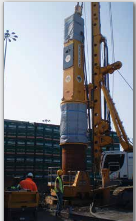
BSP CG300, with acoustic shrouding, driving tubular piles
