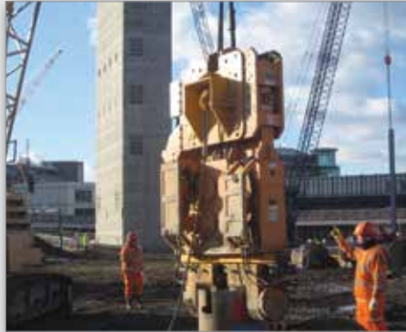
PVE 2316VM, fitted with casing handling brackets, driving tubular piles
