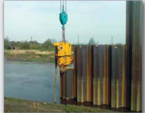
PVE 38M installing sheet piles to repair a failing sea wall
