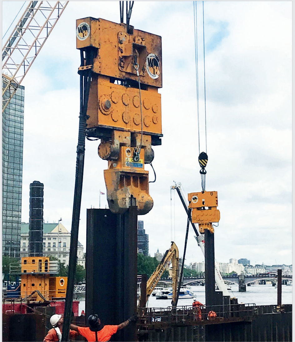
Two PVE 40VMs driving 'AZ' pairs for a cofferdam
