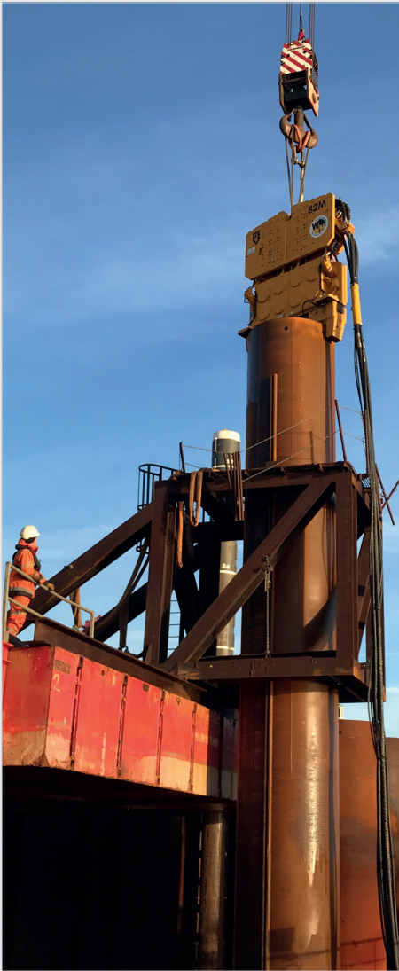
PVE 82M installing tube piles for a harbour wall
