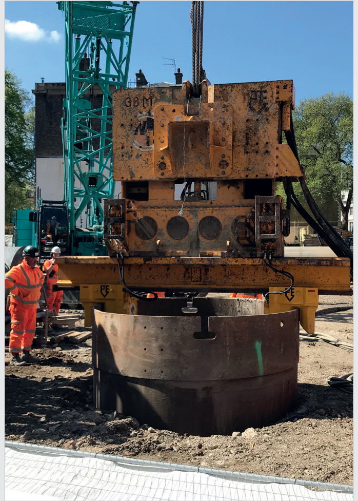
PVE 38M driving a 2.4m tube with bespoke beam and clamp arrangement
