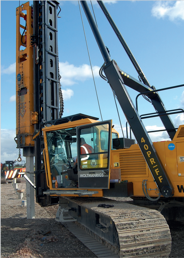
Woltman 40PR installing precast concrete piles
