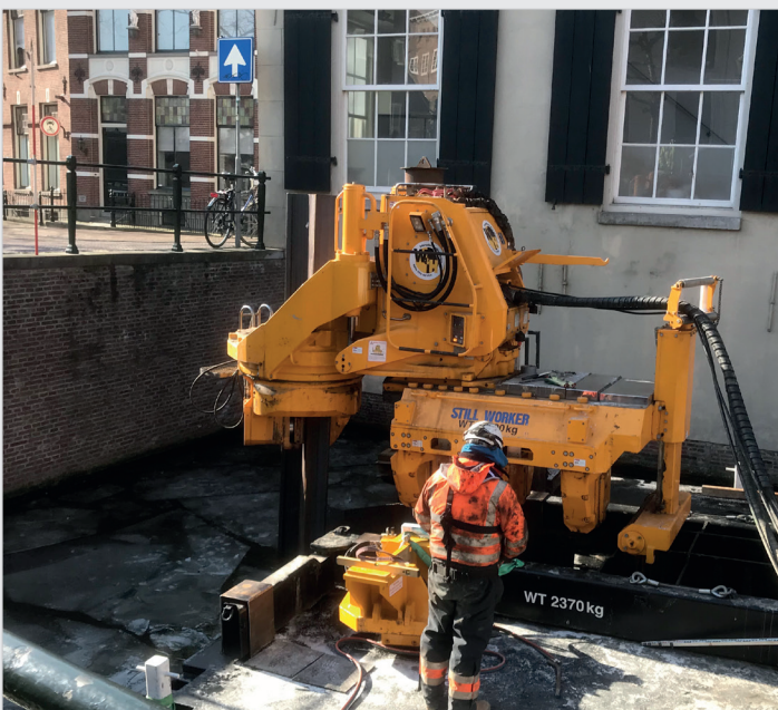
Kowan Still Worker ZU-100 pressing 'Z' piles on a canal in the Netherlands
