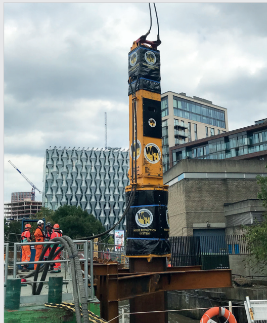
BSP CG210, with acoustic shroud, driving tube piles
