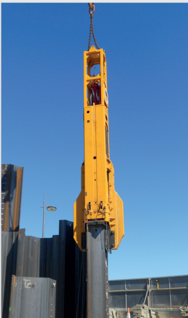
BSP CX110 with wide-cap driving 'AZ' pairs
