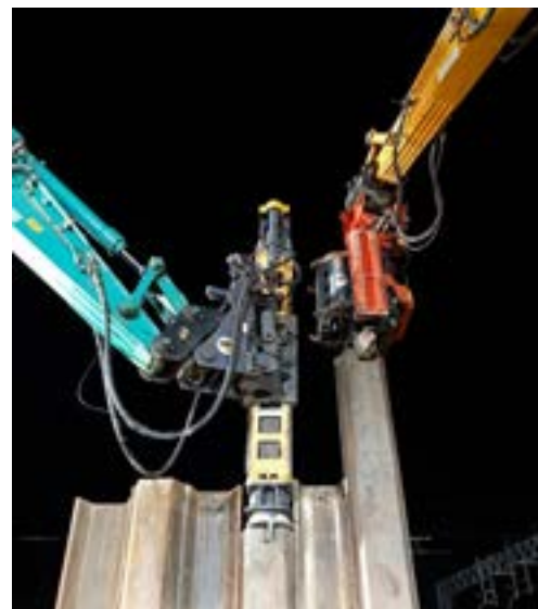
DH impact hammer and Side Grip night time rail project
