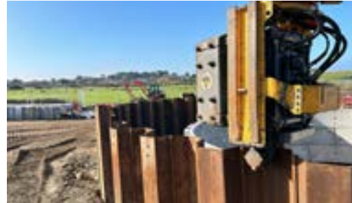
Circular cofferdam using an SG-75V Side Grip vibrator and DH-25 impact hammer
