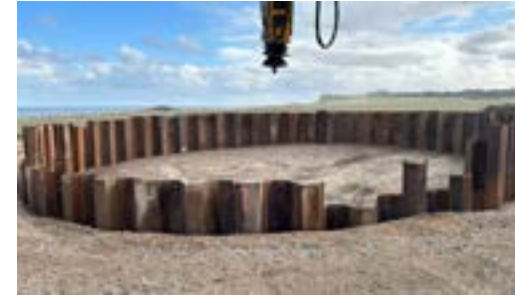
Circular cofferdam using an SG-75V Side Grip vibrator and DH-25 impact hammer
