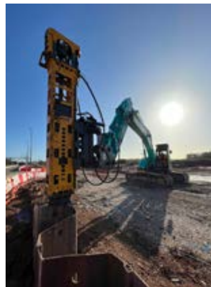
Back driving with a DH-25 impact hammer
