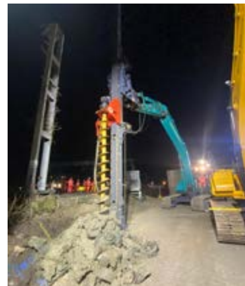
MPL-300 pre-augering ahead of sheet pile installation
