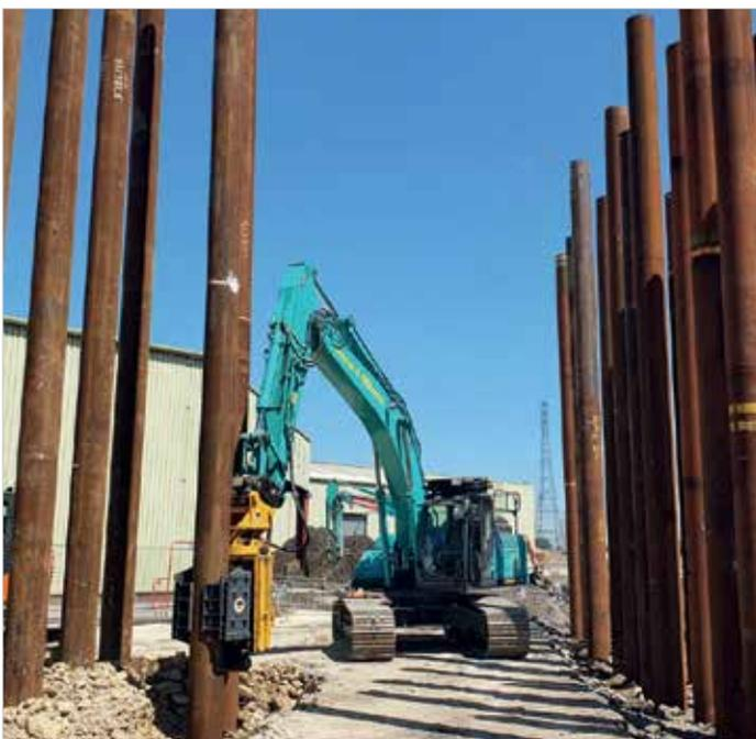
Movax SG-75V installing tube piles in Lincolnshire
