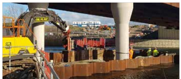
Movax SG-75V driving sheet piles under a bridge in Kent
