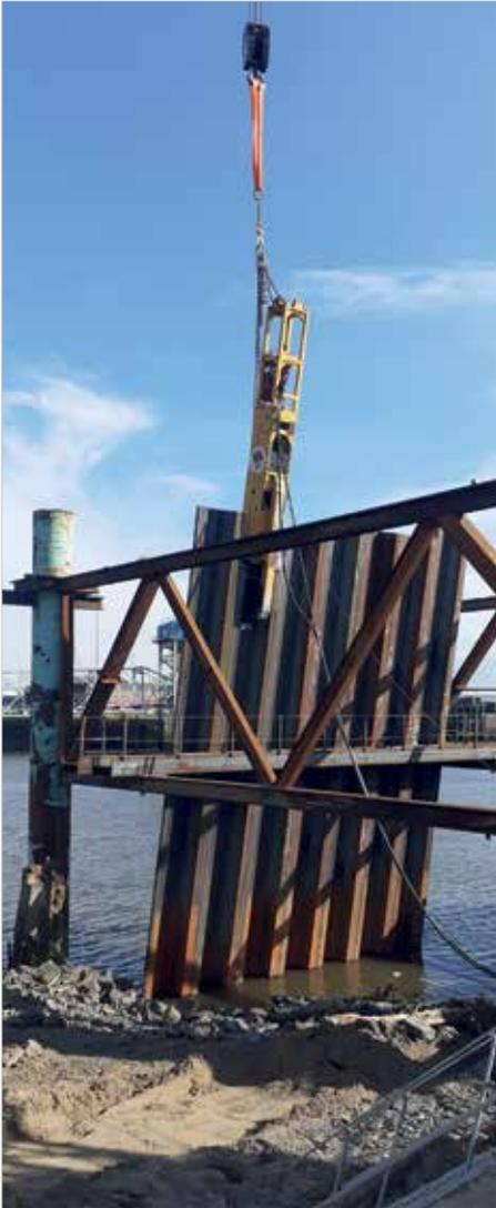
BSP CX579 driving raked sheet piles in Wales
