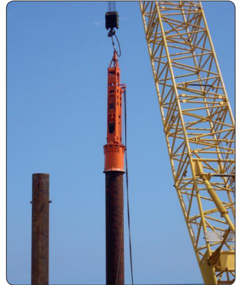
CX110, Crane suspended and fitted with tube guide
