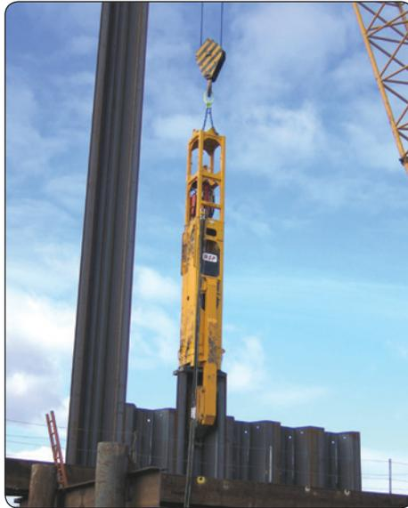
CX85, Crane suspended and fitted with legs and inserts for driving sheet piles
