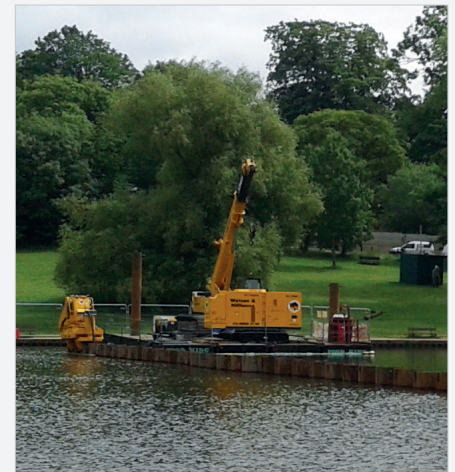
Work over water
